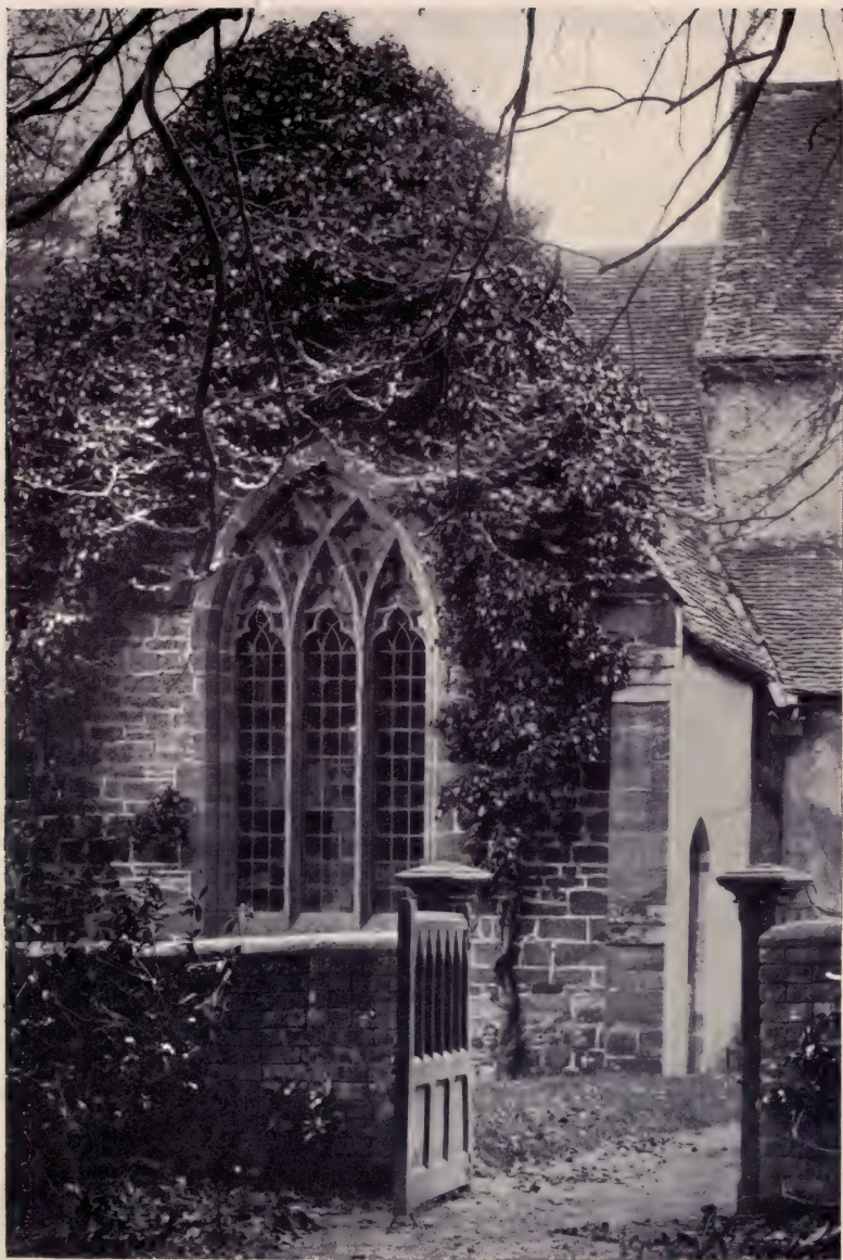
WINDOW IN THE NORTH TRANSEPT OF KINLET CHURCH
